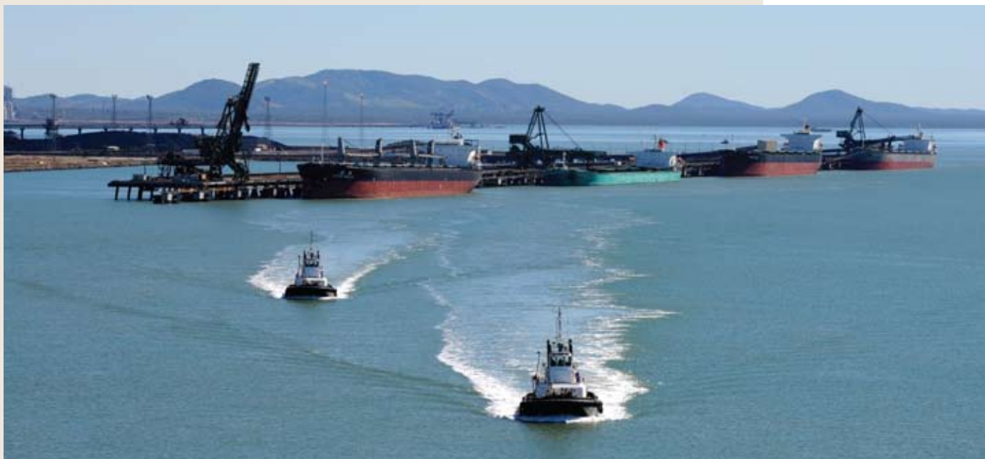
The RG Tanna Coal Terminal, Port of Gladstone, Queensland. Photo courtesy of Gladstone Ports Corporation Limited.
