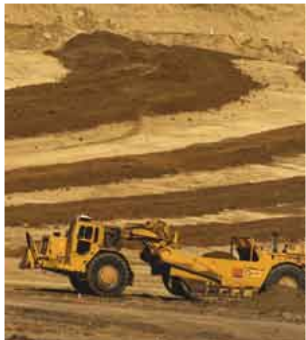
Rehabilitation in progress at Curragh.
