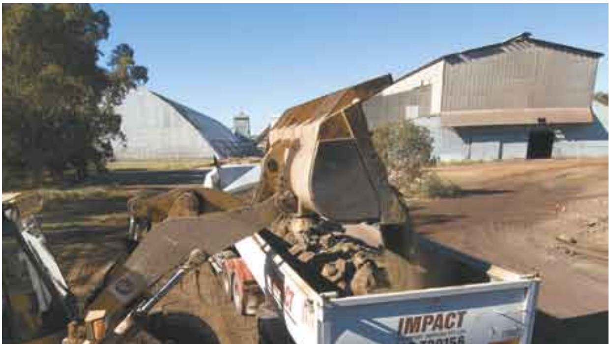
Removing soil from a contaminated site at Bayswater, Western Australia.
