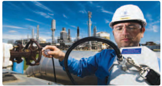
Process Operator, Mark McCafferty, carrying out a gas detection test at the Wesfarmers LPG facility at Kwinana, Western Australia.
