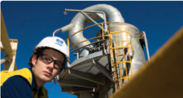
Graduate Engineer, Andrew Carruthers, at the sodium cyanide plant at Kwinana, Western Australia.
