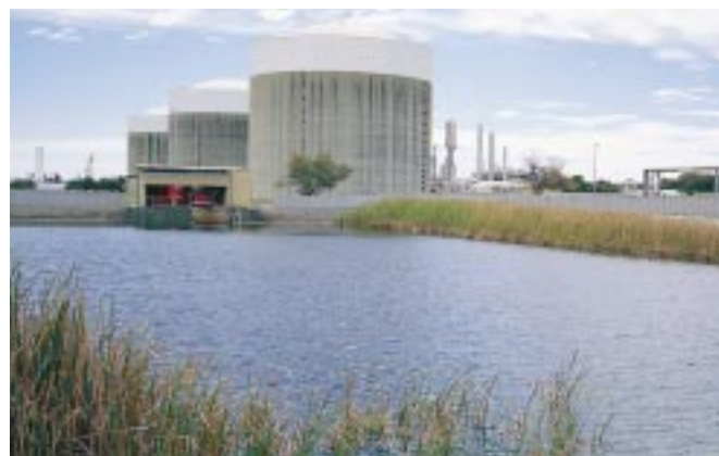
Above Export storage tanks near the dam.
