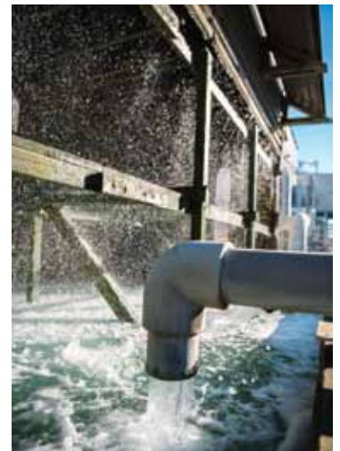
Recycled water at a cooling tower, CSBP Kwinana, Western Australia
