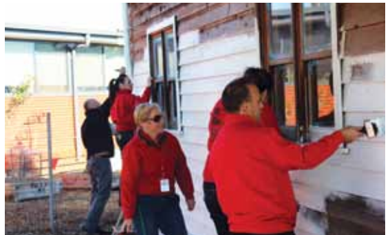
Team members painting a rundown cottage for special needs children at a school in Mickleham, Victoria
