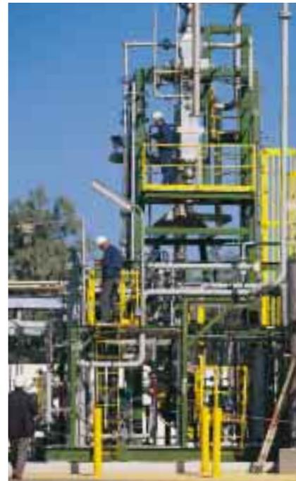
**Carbon dioxide stripping plant at Kwinana works.**
