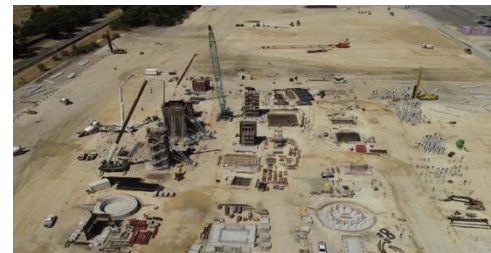
Construction of the Kwinana refinery underway.
