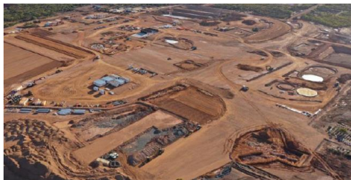
Construction of the mine and concentrator has commenced.
