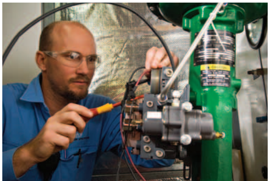
Instrument and Electrical Technician Danyul Cvitan conducting checks on an actuator valve.
