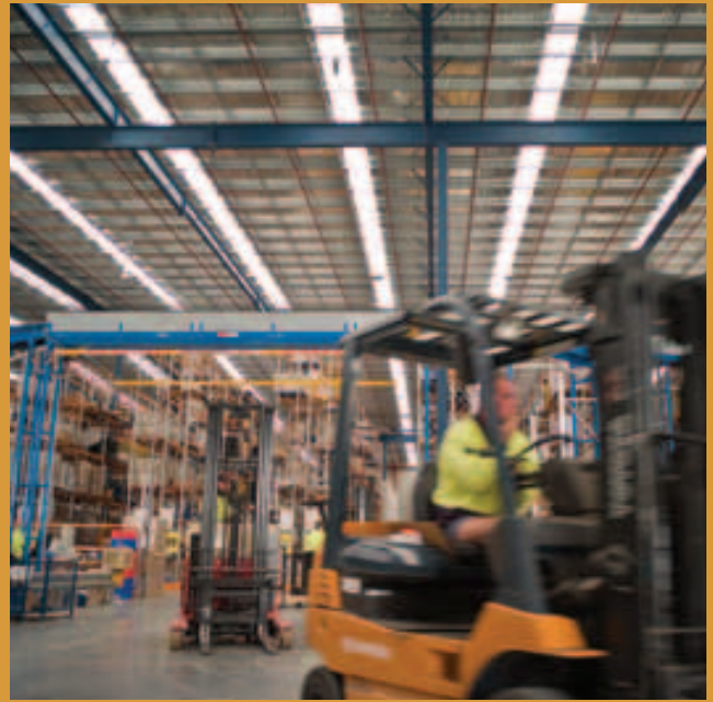
The roof of the Blackwoods distribution centre at Carole Park allows natural light into the warehouse.
