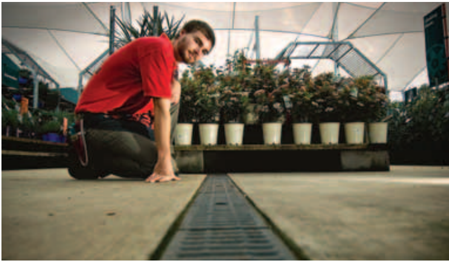
Horticulturalist Alex Mead inspects a nursery run-off recycling irrigation drain at the Stafford Park warehouse in Queensland.
