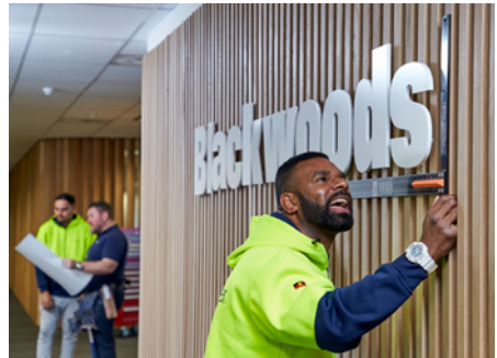
Mark Mosby, one of the tradesmen employed by Blackwoods' contractor The Builder – Sydney, puts finishing touches to the new Blackwoods office in NSW.
