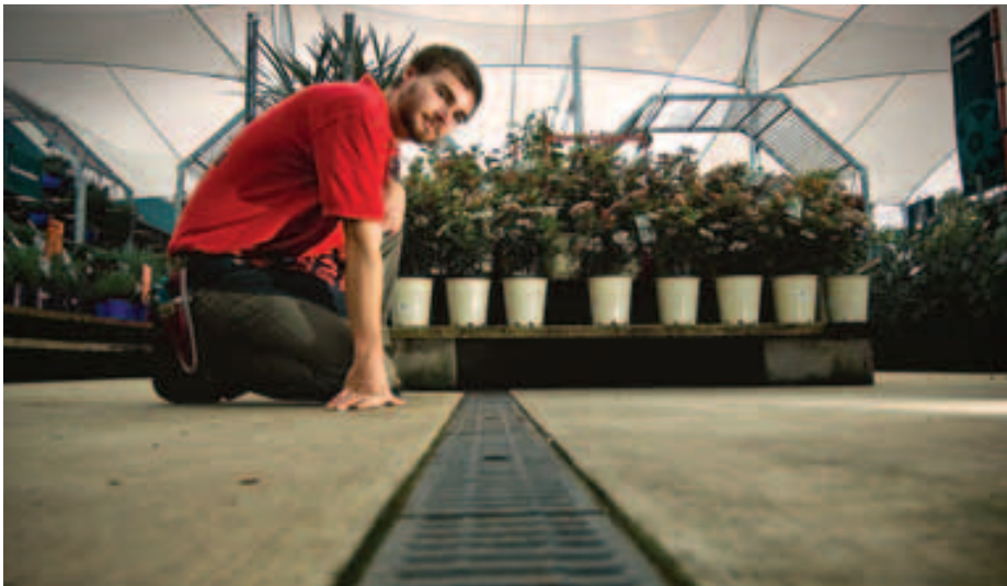
Horticulturalist Alex Mead inspects a nursery run-off recycling irrigation drain at the Stafford Park warehouse in Queensland.
