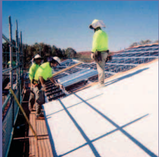
Safety Assist has helped to reduce accidents in the New Zealand roofing industry.
