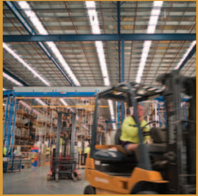
The roof of the Blackwoods distribution centre at Carole Park allows natural light into the warehouse.
