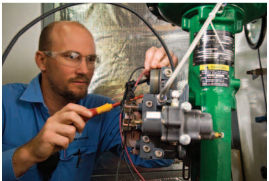
Instrument and Electrical Technician Danyul Cvitan conducting checks on an actuator valve.
