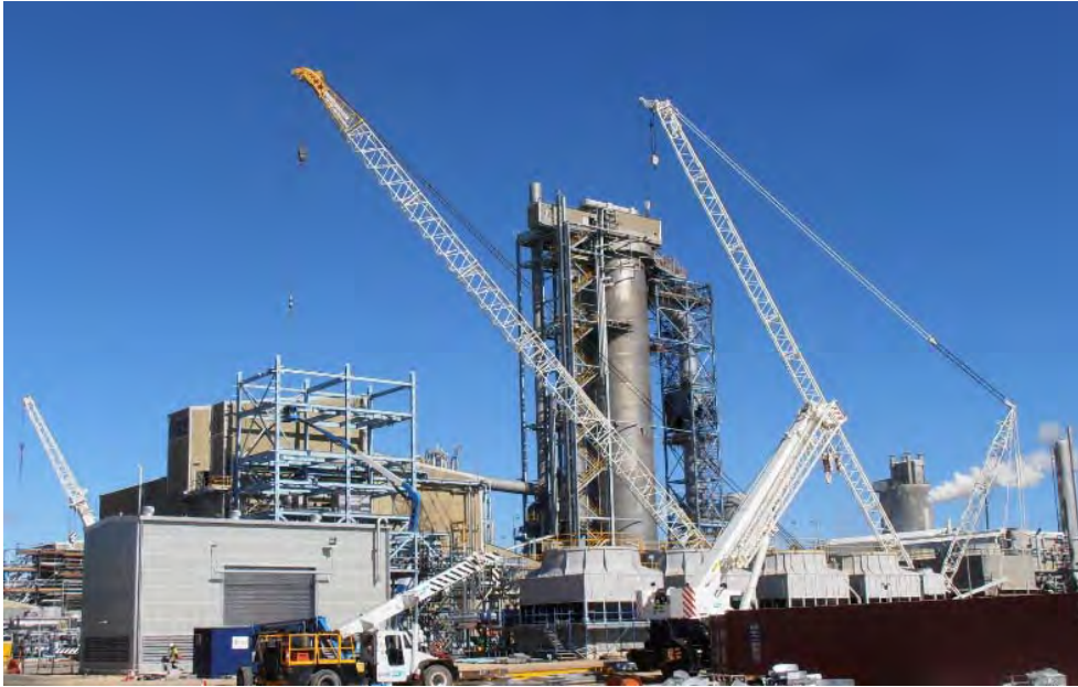
Scrubber, Prill Tower
