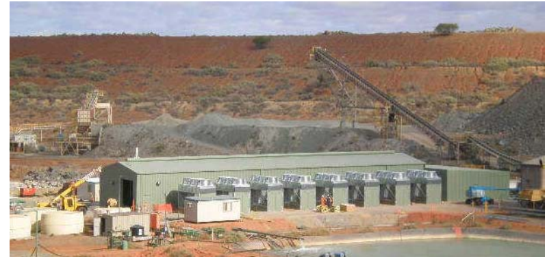
Darlot power station under construction
