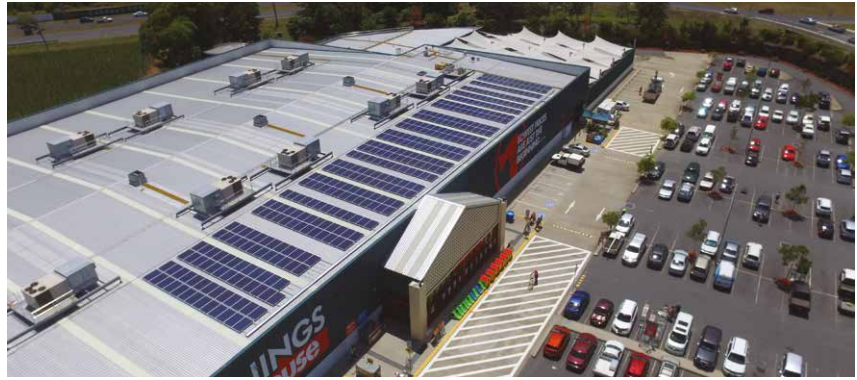
As part of ongoing efforts to improve the energy efficiency of its business operations, Bunnings has been trialling renewable micro generation projects since 2009.
